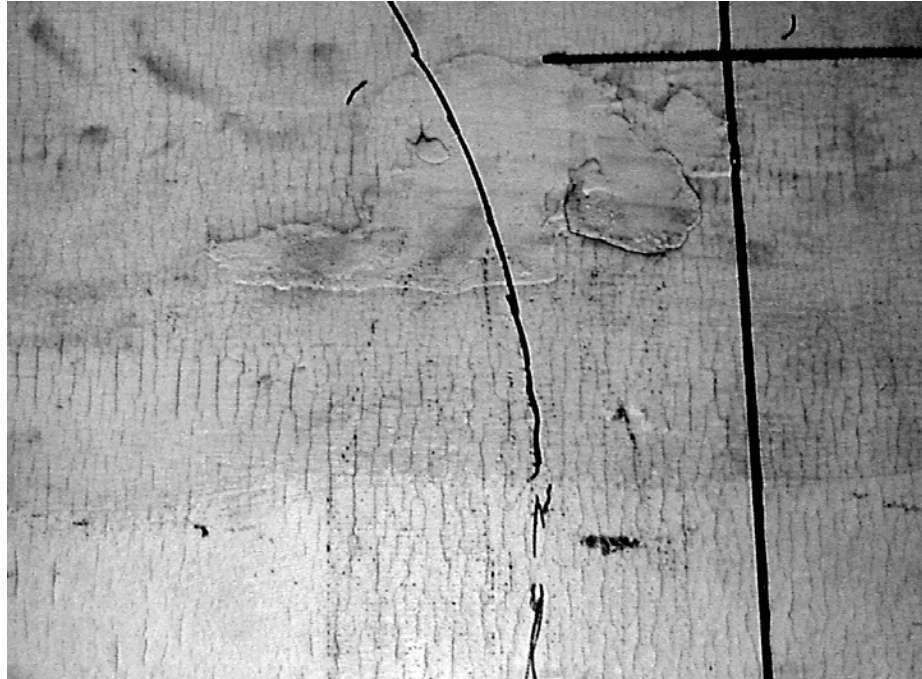
Fig. 10. Paint cracks on outside of SCV at cluster B. The curved line encloses cluster B.
